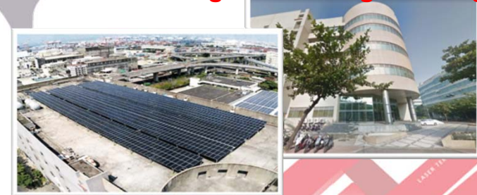
Kaohsiung Hsin Sheng Building
